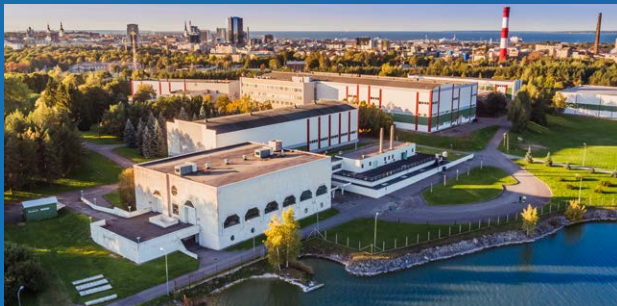
Ülemiste Water Treatment Plant
