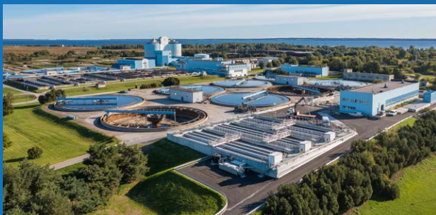
Paljassaare Wastewater Treatment Plant
